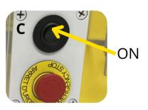
If it still doesn't work, check if the fuse of the disconnector switch ED-001 is not blown. If so, reset the Manual Resettable Fuse by pressing the button.
